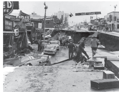
Collapse of Fourth Avenue near C Street, Anchorage, due to landslide caused by earthquake.
